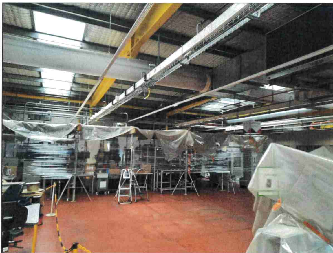
FIGURE 7 – PROTECTION DES MACHINES
